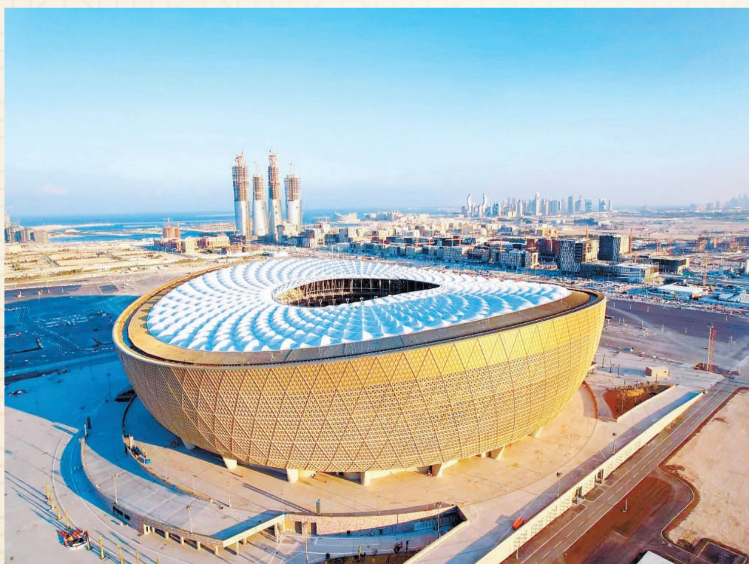
The Lusail Stadium is China's first overseas World Cup stadium construction project.
