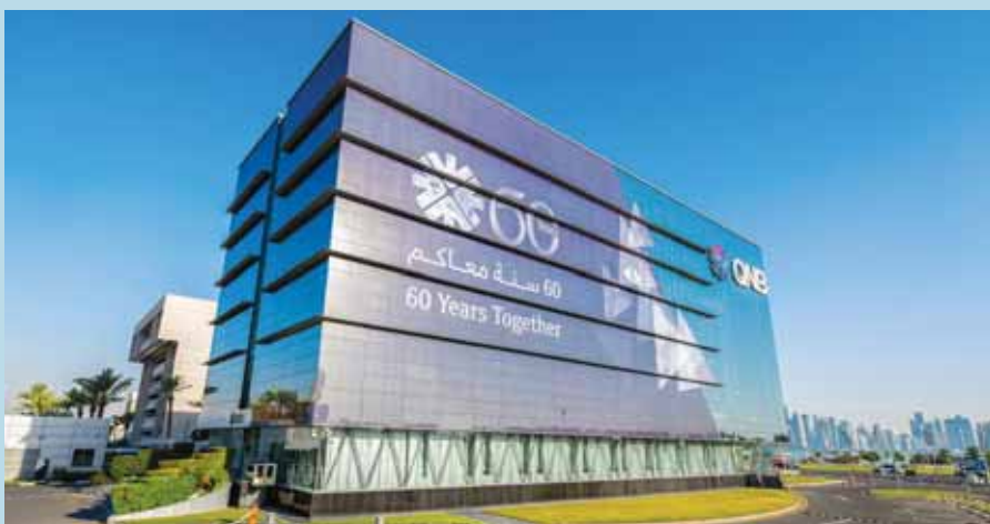
QNB's share buyback is a confidence building measure, which is expected to raise investors' trust in QNB's robust capital allocation process, improve market liquidity and enhance returns
