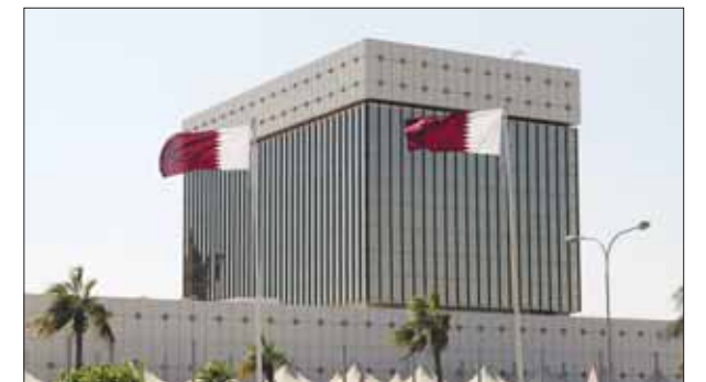
Fawran is considered one of the most innovative and advanced services, in line with the third strategy for the financial sector in the country and in continuation of the QCB's efforts to develop the infrastructure of payment systems and keep pace with the latest developments in payment systems and electronic transfer of funds. Fawran was designed in accordance with a system based on the latest technologies and security standards, to maintain the security and confidentiality of the information created by the QCB to enable financial institutions to provide the service to their customers with complete reliability
