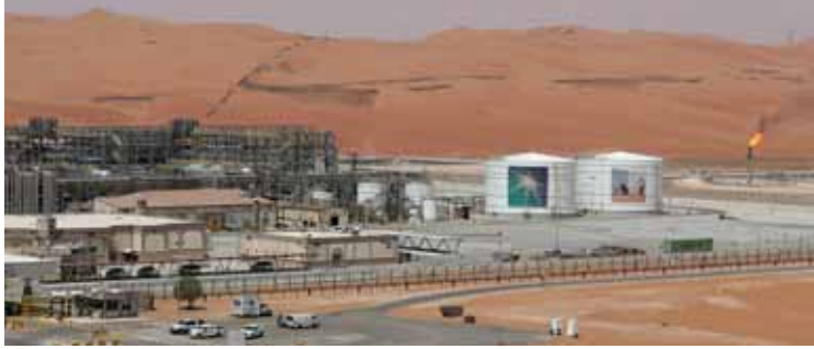
A view of the production facility at Saudi Aramco's Shaybah oilfield in the Empty Quarter. Economic growth in Saudi Arabia will accelerate next year thanks to higher oil output after two years of modest performance, according to a Reuters poll of economists, who also forecast robust growth for other GCC states.
