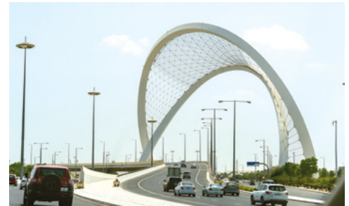
The Lusail Expressway project involves the construction of expressway running from central Doha to the Pearl area. The 100-meter-high huge arches are the landmark on the way from Hamad International Airport to Lusail Iconic Stadium.
