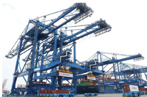
The Pier 7, Busan New Port, showing the growth on exports.
