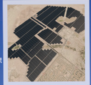
QEIC Solar Project
