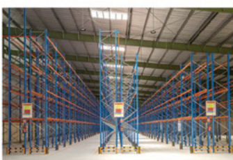
Selective Pallet Racking
