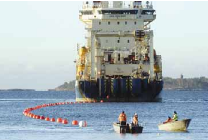
This file photo shows C-Lion1 submarine telecommunications cable being laid to the bottom of the Baltic Sea by cable ship Ile de Brehat on the shore of Helsinki. (Reuters)
