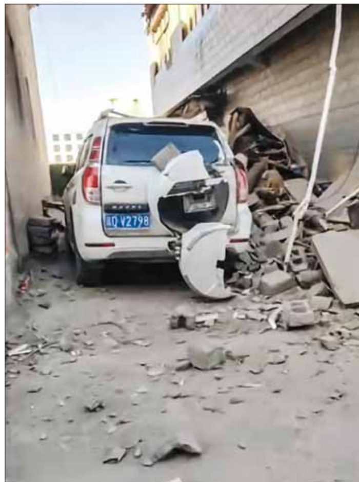
Damage in Lhatse County in Shigatse city in China's Tibet.
