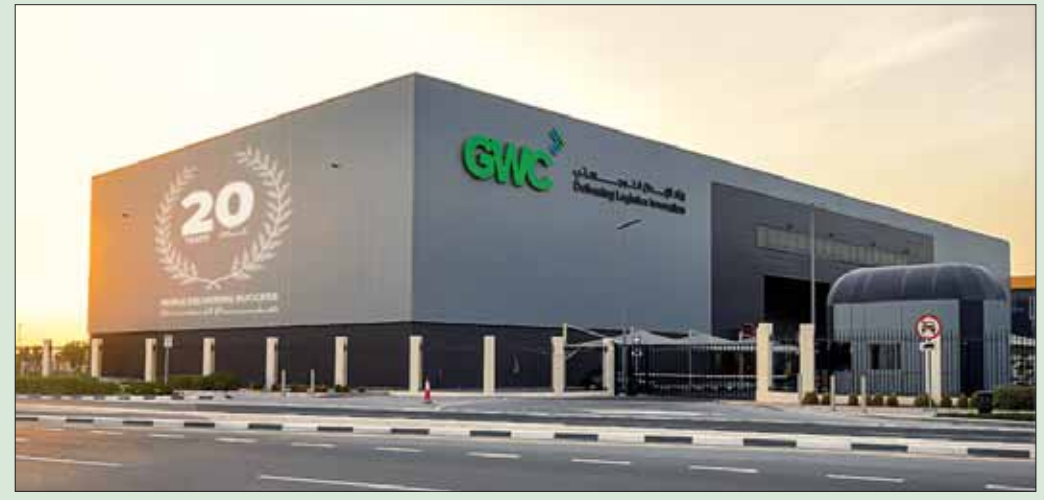
GWC's facility at Ras Abu Fontas Free Zone.
