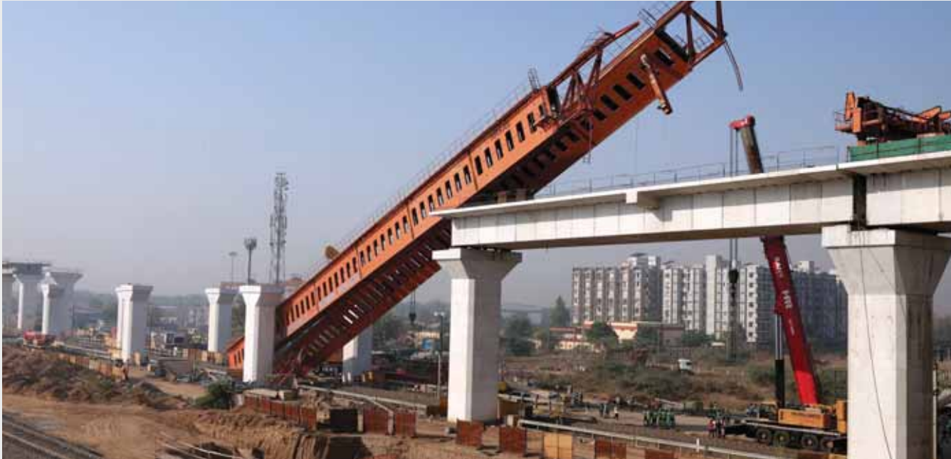
Employees of National High Speed Railway Corporation Ltd work on restoration after a slab-launching crane collapsed between two pillars near a massive gantry that was being used to install concrete girders between pillars on the Ahmedabad-Mumbai bullet train project, on the outskirts of Ahmedabad, India, yesterday.
